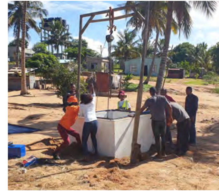
Mozambique – In Quissico, a defective submersible pump that needs to be replaced is lifted from a pump well. Photo taken by Short Term Expert Paul Bruggeman.
