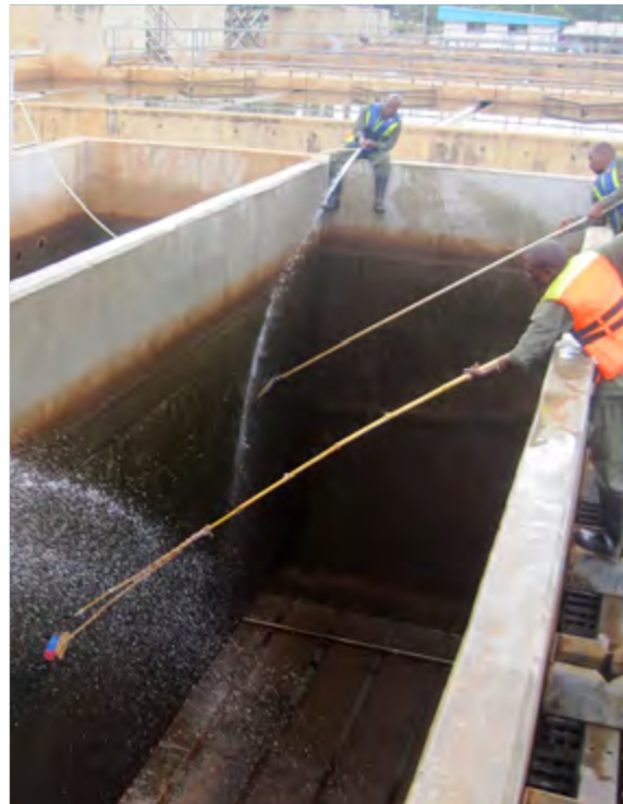
◀ Malawi – Cleaning of the sedimentation tanks of Treatment Plant 2 at Lilongwe Water Board. Photo taken by Short Term Expert Kees Hagen.
