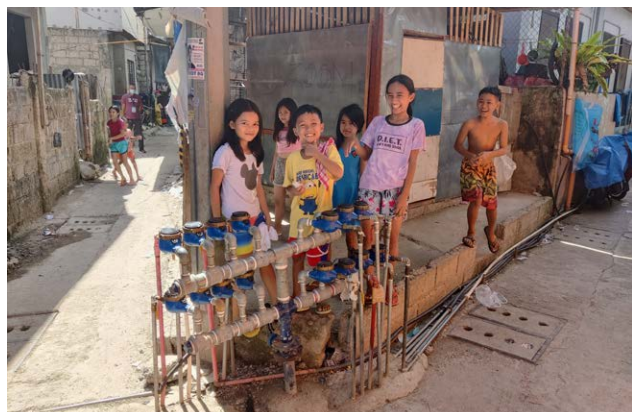
Sitio Tahna (before and after): overloaded stub-outs with spaghetti pipes were replaced with expansion pipes and extended stub-outs into the heart of the community
