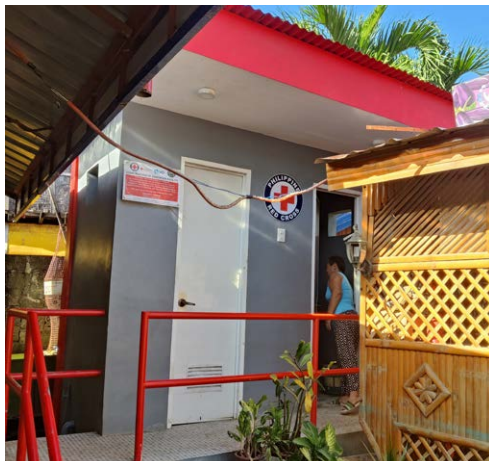
Tanke, Talisay City Maintained latrine
