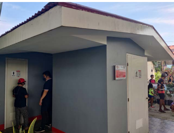
Cebu city Communal latrine facility
