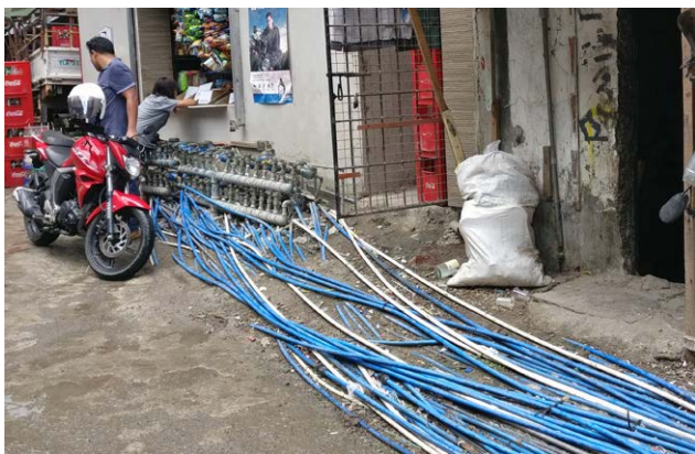
Sitio Tahna (before and after): overloaded stub-outs with spaghetti pipes were replaced with expansion pipes and extended stub-outs into the heart of the community
