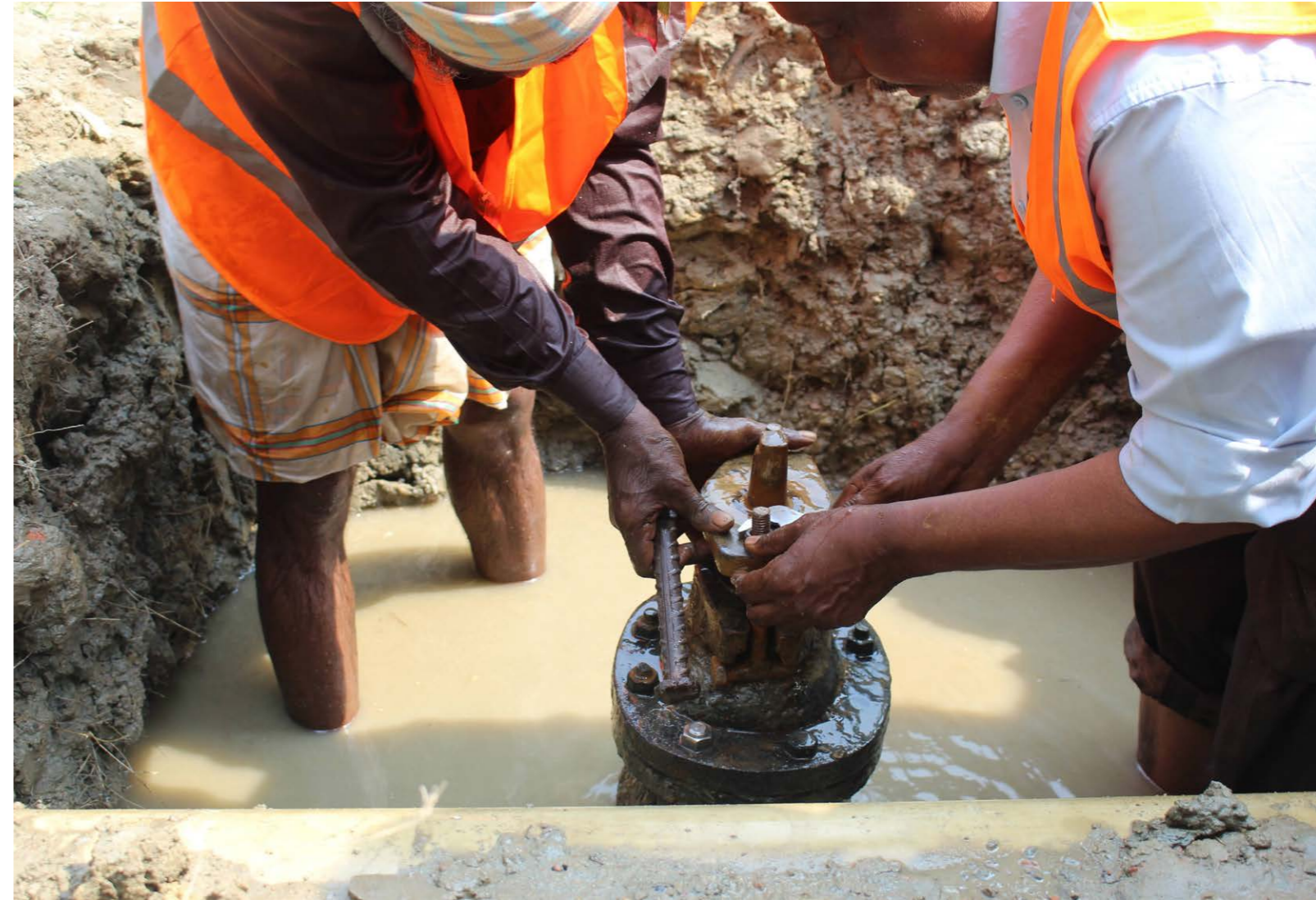
Bangladesh – Dhaka WASA plumbers are repairing a valve, 2020.
